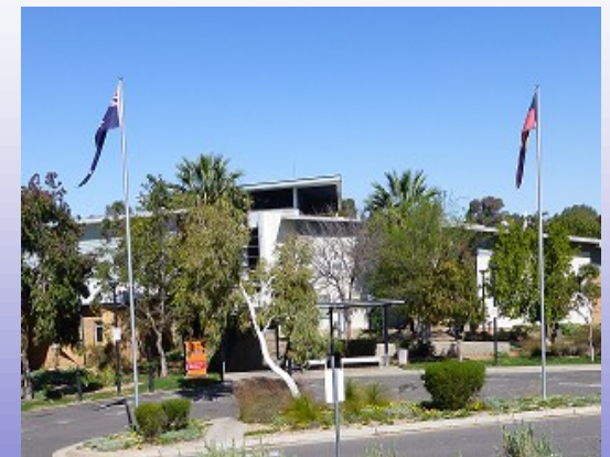
Broken Hill Hospital
